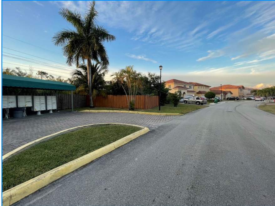
Figure 8: Missing pedestrian connectivity
