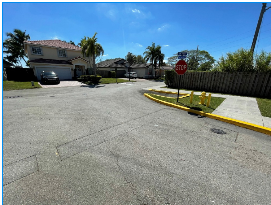
Figure 7: Missing stop bar markings
