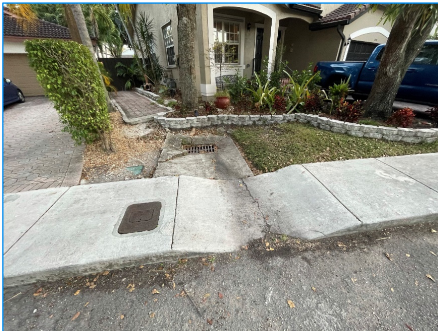
Figure 9: Depressed sidewalk
