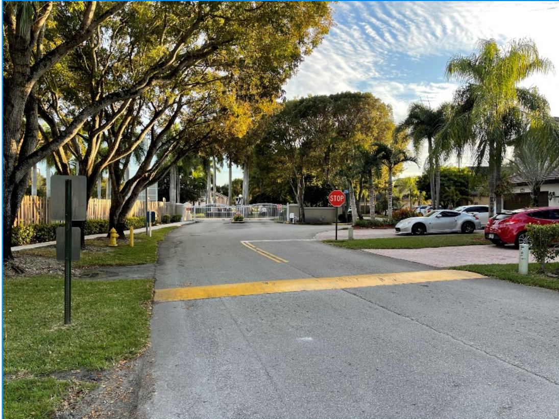
Figure 6: Speed bump installed too close to intersection
